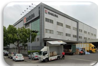
Daya plant II Water heater · Gas stove
